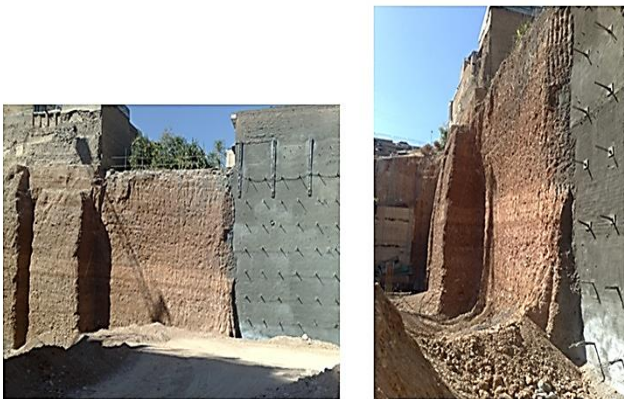
Fig. 1. Investigated wall of excavation site (west-side wall).
