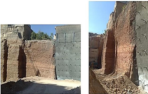
Fig. 1. Investigated wall of excavation site (west-side wall).
