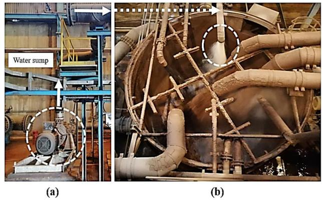
**Figure 10.** The dilution pump (a) and dilution tank (b)
