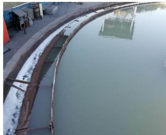
**Figure 11.** The thickener surface after modification in the operation condition
