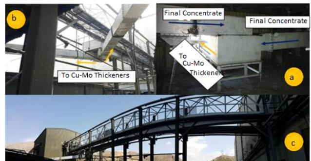
Fig. 4- Combining final concentrate of two sections (a), dividing the concentrate between two Cu-Mo thickeners (b), overall view of the gravity transportation channel (c).
