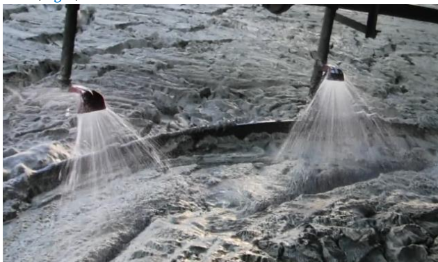
Fig. 6. Modifications applied on the feedwell to break the froth.
