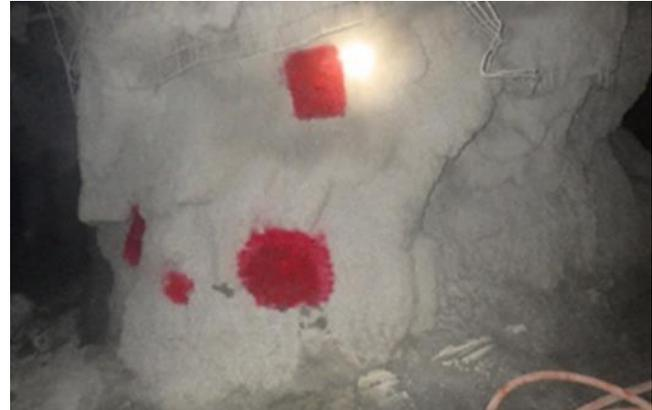
Fig. 35. In-stope with no damage after seismic events took place.
