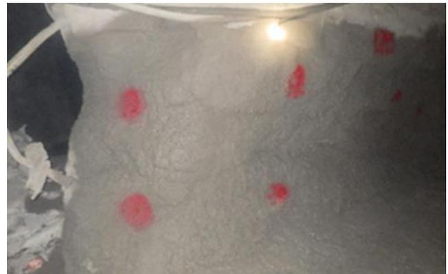
Fig. 36. In-stope with no damage after seismic events took place.
