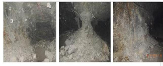
Fig. 28. Damage noted within the de-stress cuts after seismic events within the de-stress cut.
