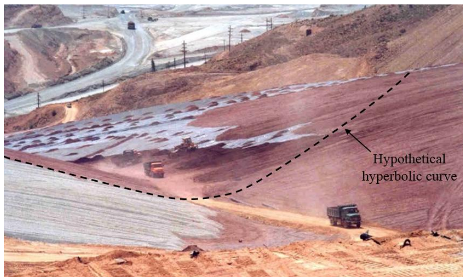
Figure 4. Hyperbolic shape of heap leaching structures foundation (Valley 2, Sharcheshmeh 2 heap leaching structure)
