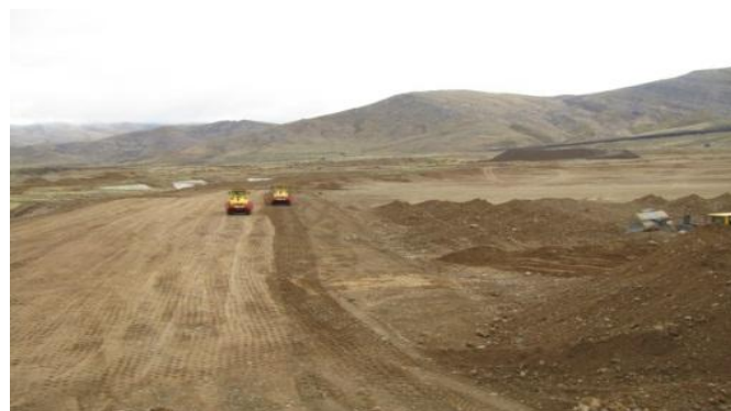
Figure 11. Foundation of Tarom heap leaching structure.
