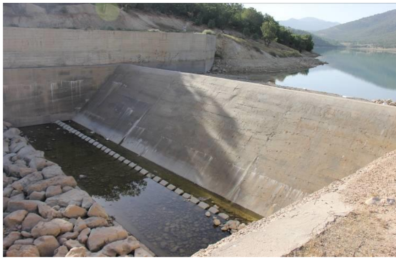
Fig. 1. a) Ogee spillway of Shahghasem dam
