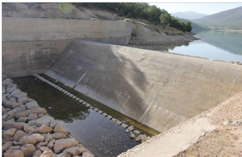
Fig. 1. a) Ogee spillway of Shahghasem dam
