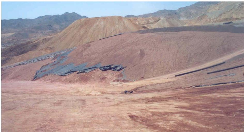
**Figure 2. Isolated layers of Sarcheshmeh copper heap leaching structure 2**
